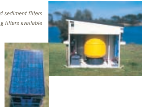
roof of unit showing the solar panel
